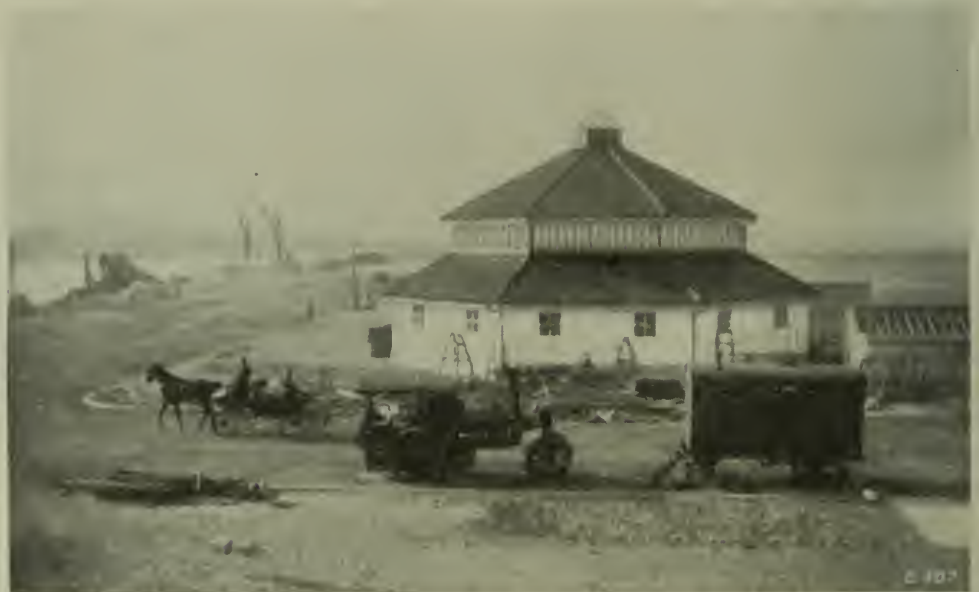
FIG. 3. THE FISH MARKET AFTER COMPLETION.
